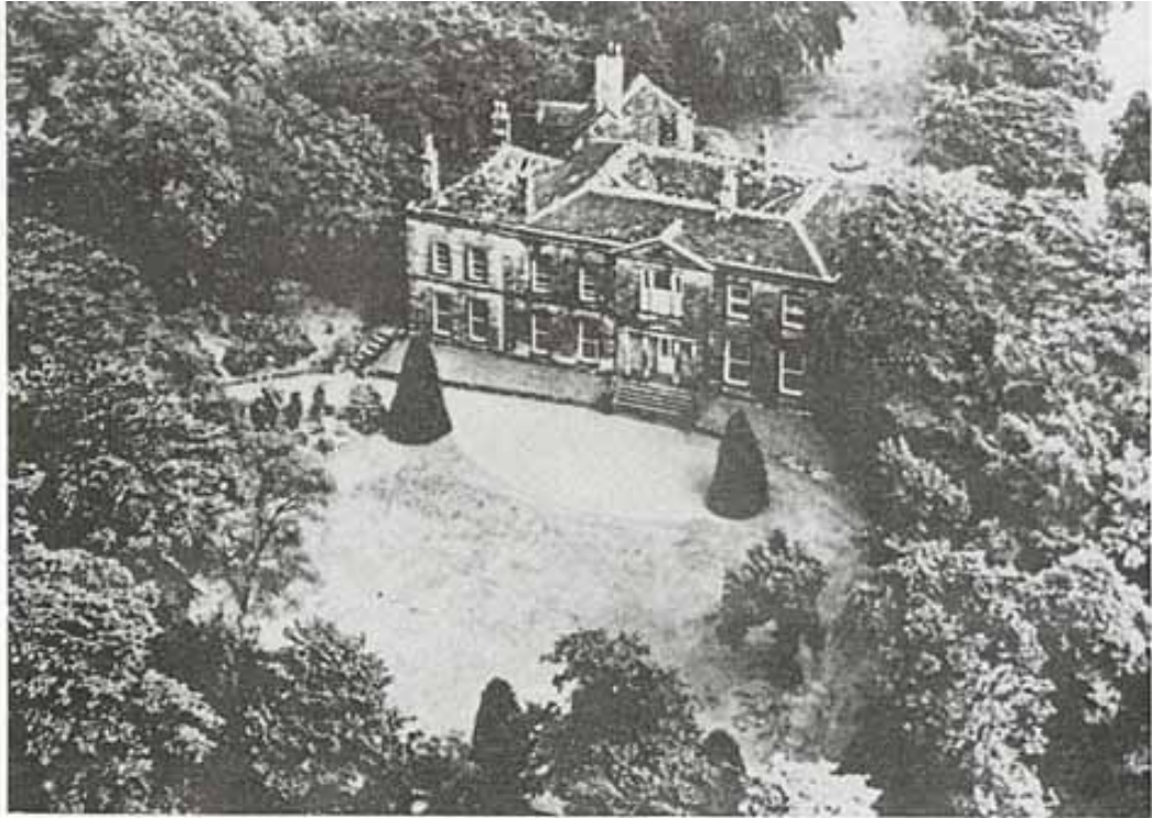
Above: the eighteenth-century hall built by the Walkers on the site settled by the Lascelles family c 1175.
