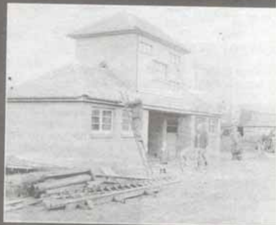
REPAIRS: Workers improve the pavilion at Bradley Mills Cricket Club in the 1950s
