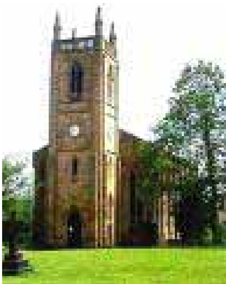
St. Paul's Church, Hanging Heaton
